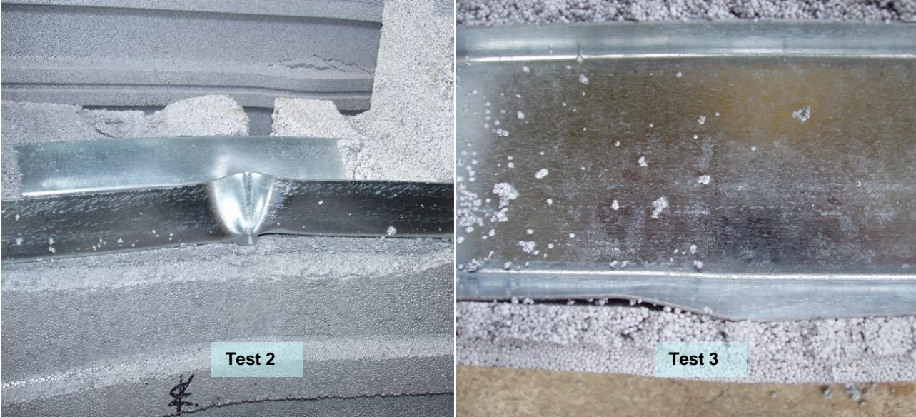
Figure 13. Buckling in the compression flange of steel 'C' profiles.
